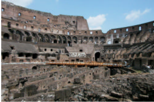
Figure 2 : The rebuilt arena in line with the hypogeal masonry structures
