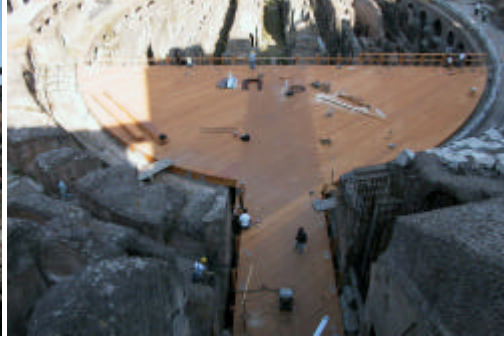
Figure 3 : The rebuilt arena and the eastern entrance corridor
