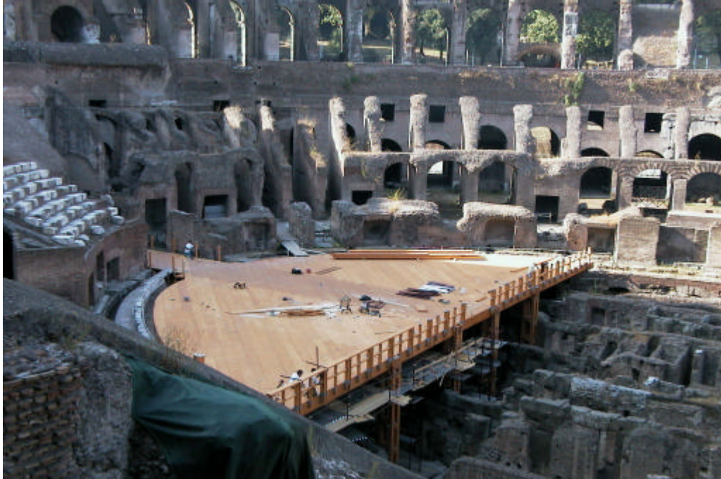
Figure 1 : The arena flooring rebuilt by laminated wood at the Flavian level
