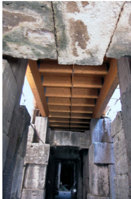
Figure 5 : Timber structures of the entrance corridor leaned on interposed blocks.
