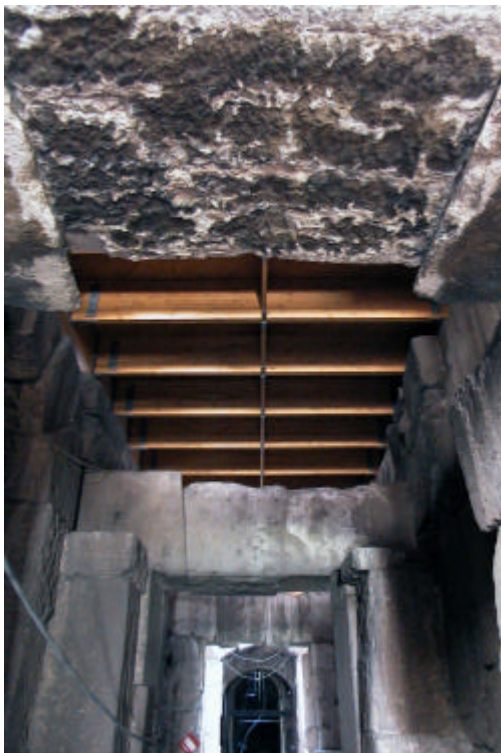
Figure 6 : Timber structures of the entrance corridor directly leaned on the travertine blocks
